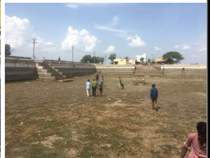
The image of pond after cleaning (08.08.2017)
